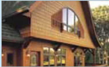
Fiber Cement Siding
